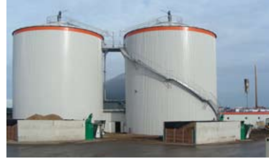
High upright digester
