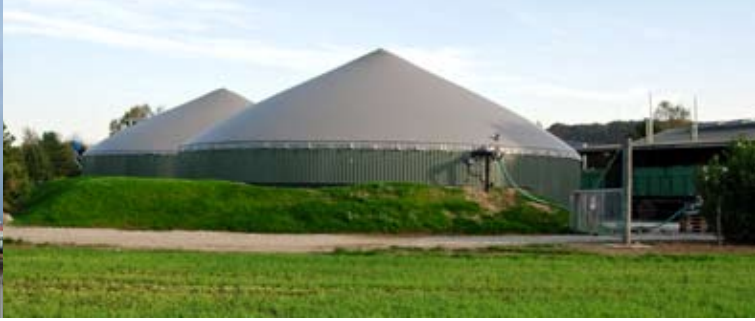
Flat digester with gas holder roof
