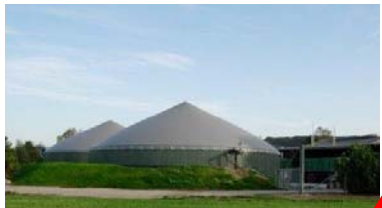
Kitchen Waste Digestion
