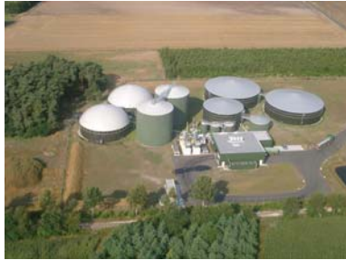
Central Biogas Plant
