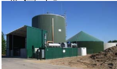
Energy Crop Biogas Plant
