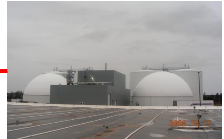
Biogasanlage Prince Edward Island
